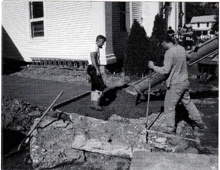
Pouring the Front Entry Walk
