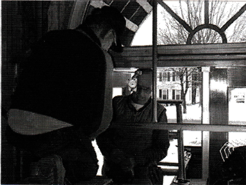
Dick vonBergen & Bill Waldruff Working on New Doorway
