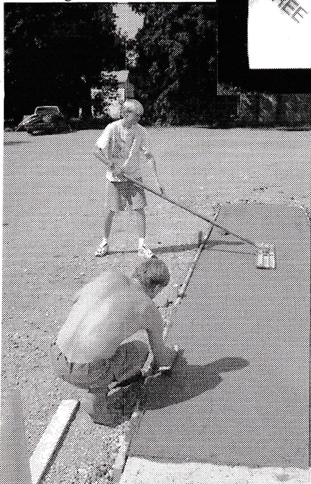
Dan & Elijah Finishing Concrete
